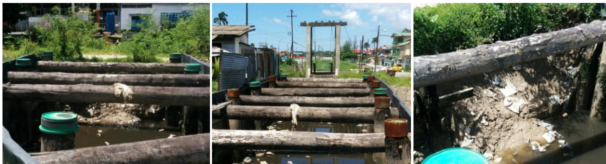
Figure 58 Silted up adjusted koker of Houston North (Joost Remmers, August 2016)
