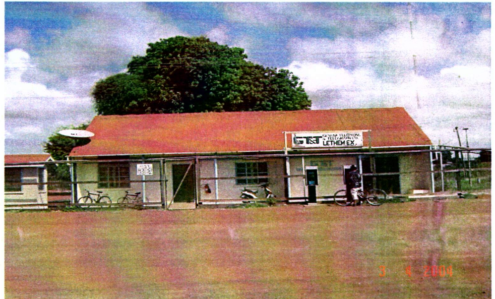
The Guyana Telephone & Telegraph Company, Lethem
