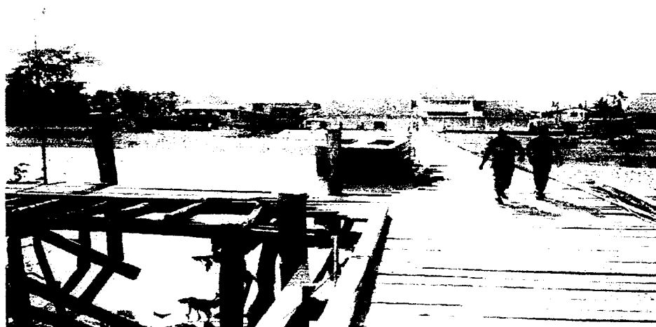
Poor state of waterfront infrastructure
