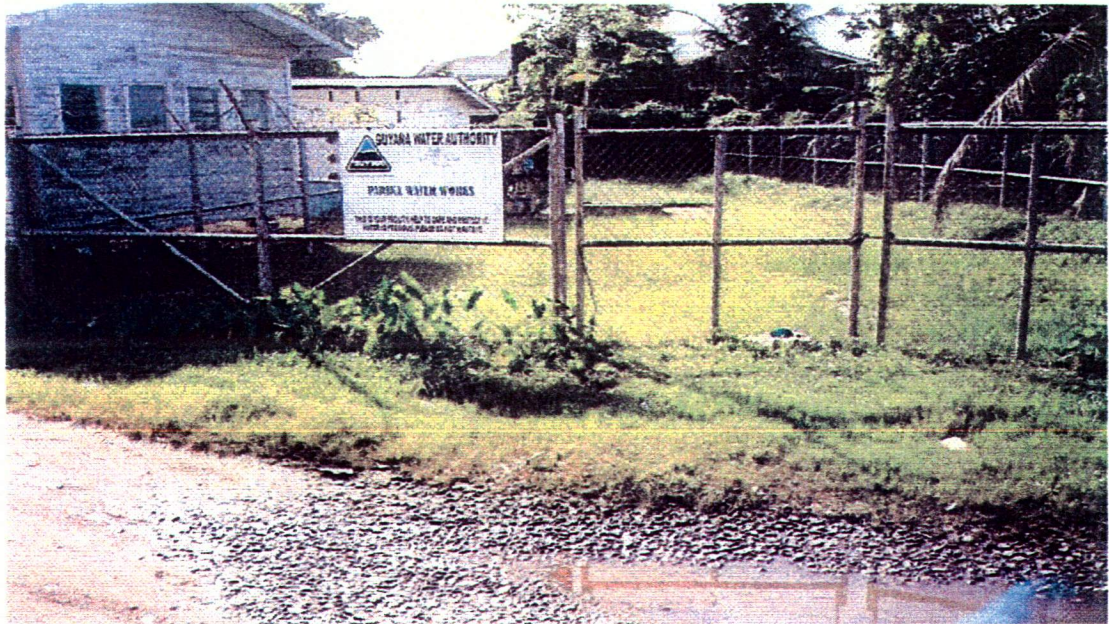
Site of the Guyana Water Authority (Serving the Parika area)
